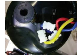
Check whether the compressor wires are properly connected with U, V, and W.
