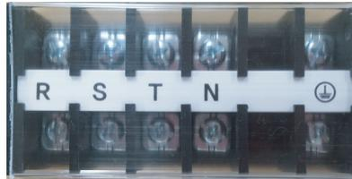
\* Compressor wire connector connection
