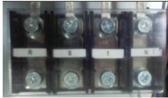
\* Compressor wire connector connection
