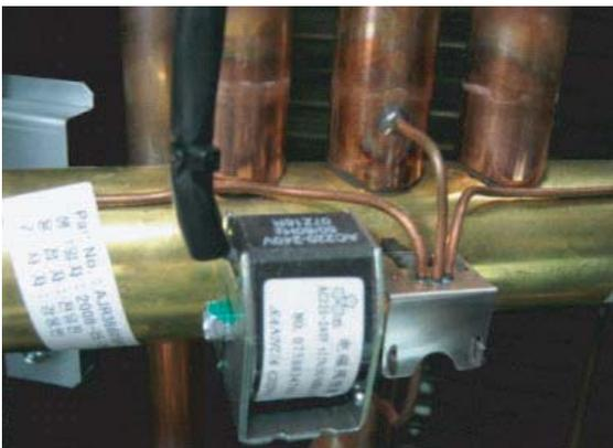
\*\*\*\* Check the output voltage of terminal socket during heating operation
