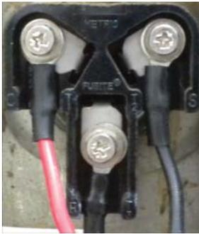
\* Compressor wire connector connection point
