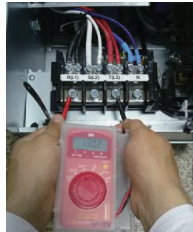
* Measuring input voltage
