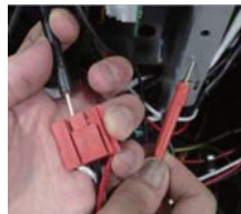
Measuring insulation resistance between fan terminal & chassis
